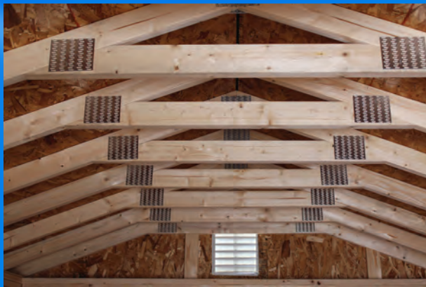
STANDARD RAFTERS 16" on Center with Stamped Truss Plates
