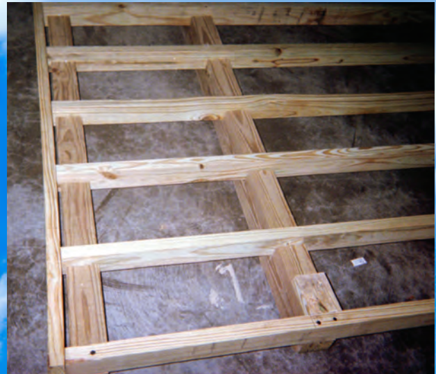
STANDARD FLOORS - Treated 4x6 Skids Notched with Treated Floor Joists 12" OC
