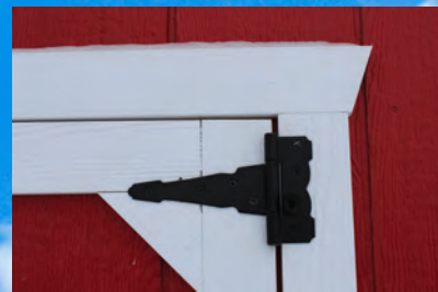
STANDARD 6" Heavy Duty T Hinge with Nylon Bushings
